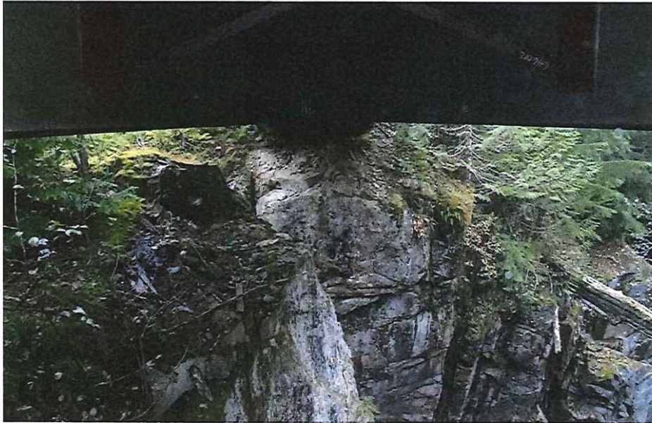
CK2122 Right Abutment
