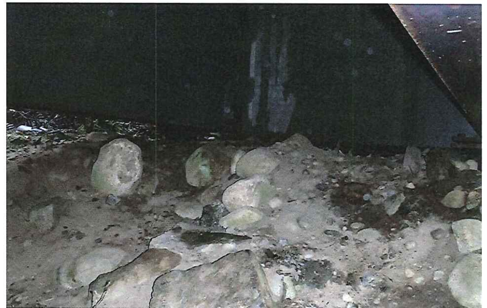
CK2122 Left Abutment
