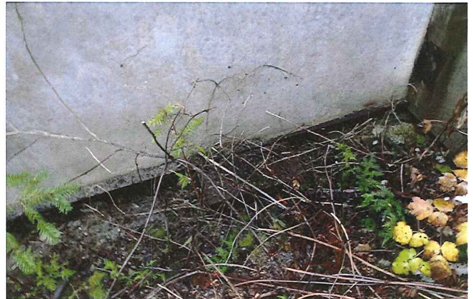
CK2122 Left Abutment Bearing
